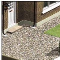
Gravel driveways and paths
