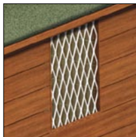
Internal diamond mesh grille over shed window
